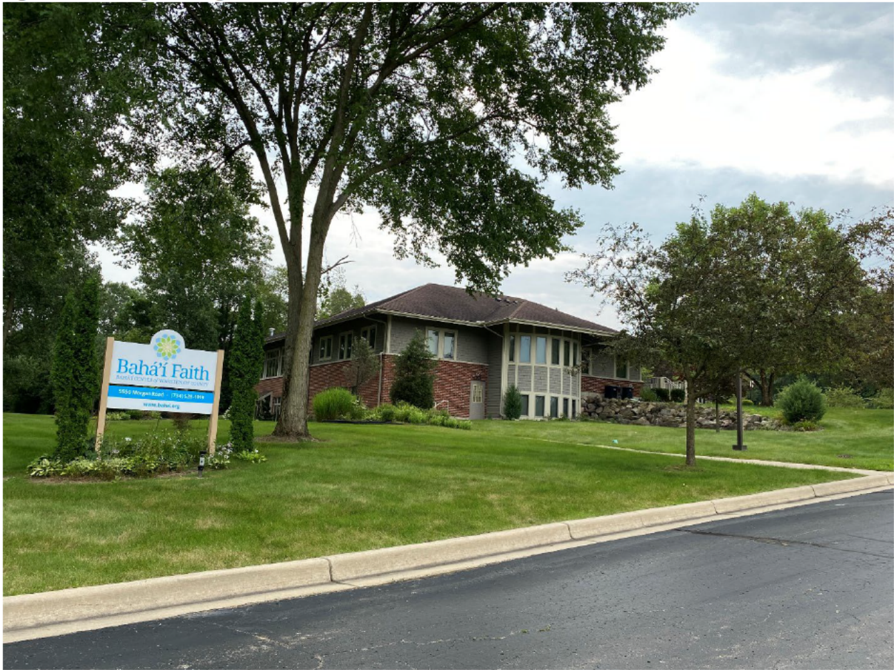
Figure 2: Existing Building – Seen from Entry Drive
